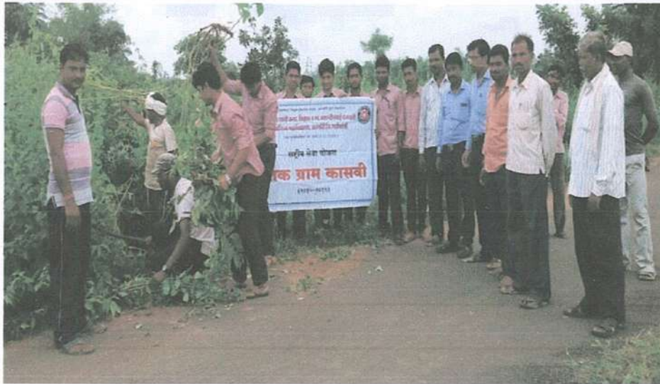
Pruning of road-side overgrown branches for clear vision of the Kasvi road
